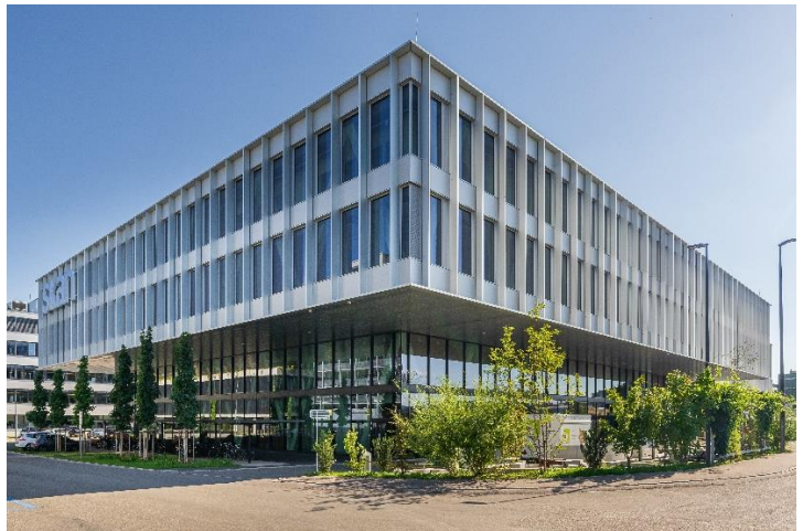
Fig. 28: Head office of SKAN AG, Allschwil (Basel)
